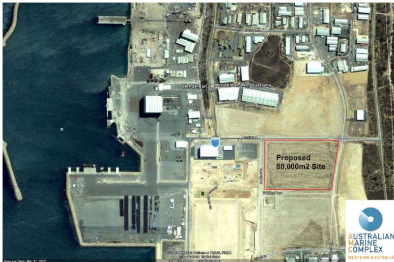
The Australian Marine Complex Site
