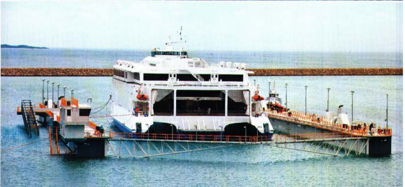
Austal using the AMC floating dock to undertake hull cleaning of its new 102 metre trimaran
